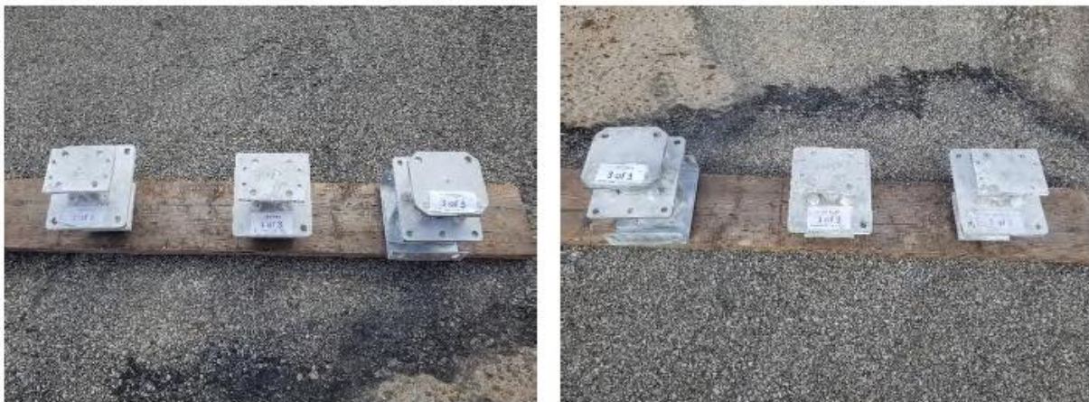
Figure 4: Water Ingress Pre-Test Condition
