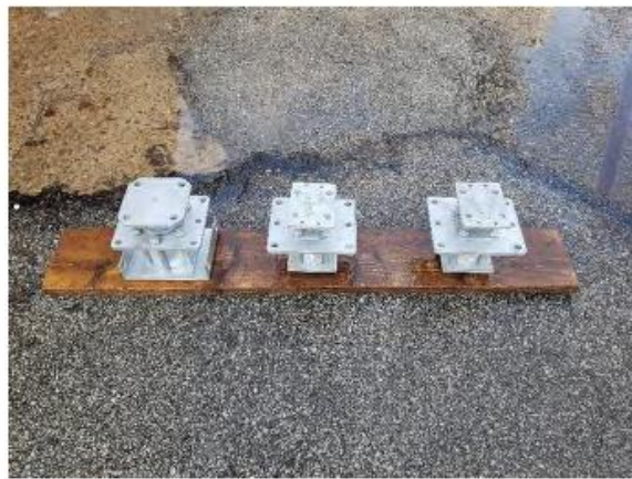
Figure 6: Water Ingress Post-Test Condition
