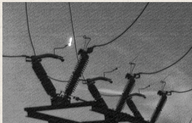
Shown is a typical line charging interruption using the Superwhip™. The whips interrupted the circuit without a re-strike. The arcs were fully extinguished within 8 milliseconds.
