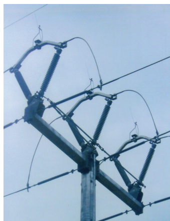
The Superwhip™ on a 138 kV CB-AV switch
