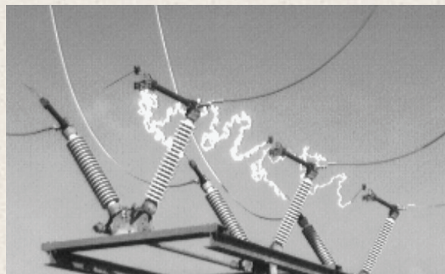
The above photo is of an actual line charging interruption event on a 115 kV circuit using a traditionally designed whip. During the switch opening there were eleven re-strikes because the whip was too slow. The photo below shows the typical difference using a Superwhip™ interrupter.
