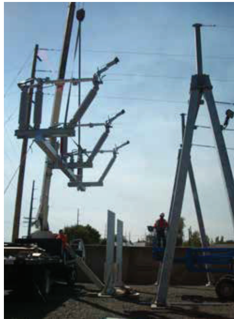
The switch is lifted into place.
