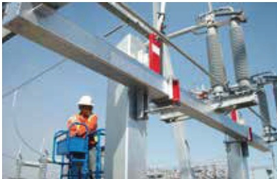
The unitized switch is attached to the supports.
