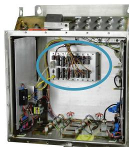
The RTU3200 in a submersible enclosure monitoring current on all phases of 10 circuits (30 analog inputs).
