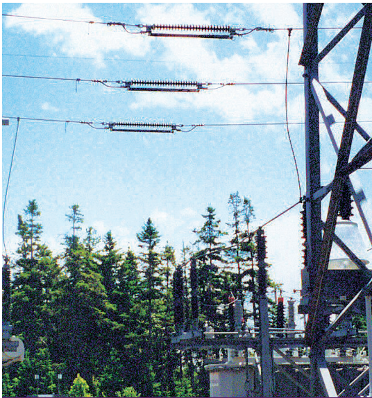
Add a sectionalizing function within the substation where space is limited.
