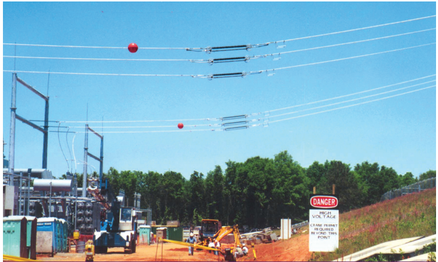
Add switches to disconnect incoming lines at a substation. 230 kV application shown.
