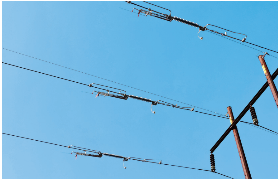
Install the ILO-C with Superwhip™ to sectionalize a transmission line and drop line charging current. 115 kV switch in the open position shown.
