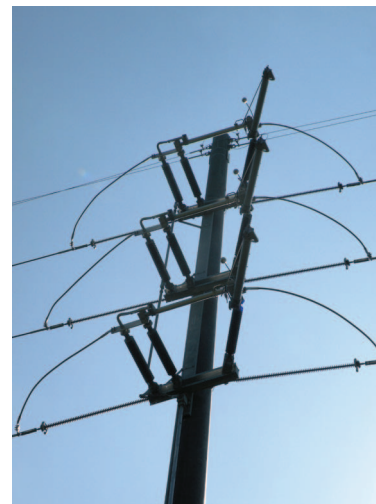
115 kV "Quick Install" vertical break switch with vacuum interrupters for full load break.
