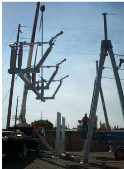
The switch is lifted into place.
