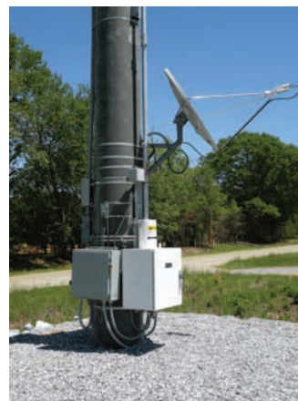
SCADA installation with BT-T motor operator and communication by satellite.
