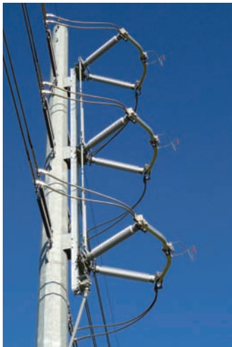
138 kV, 3000 A. “Quick Install” center break switch with porcelain insulators and quick break whips, mounted on a steel pole.
