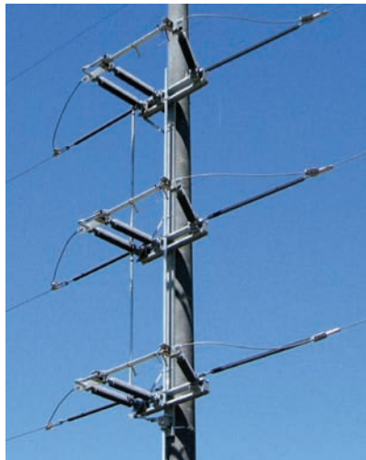
115 kV “Quick Install” vertical break switch with polymer insulators and quick break whips, mounted on a concrete pole.
