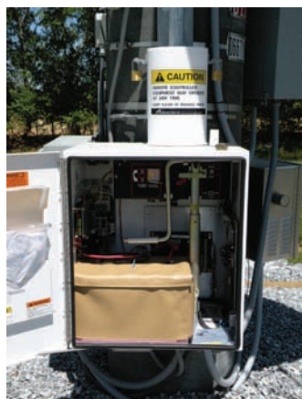
BT-T motor operator
