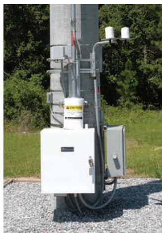
SCADA installation with BT-T motor operator and communication by radio.
