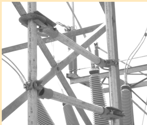
Automatic positioning mechanical interlock
