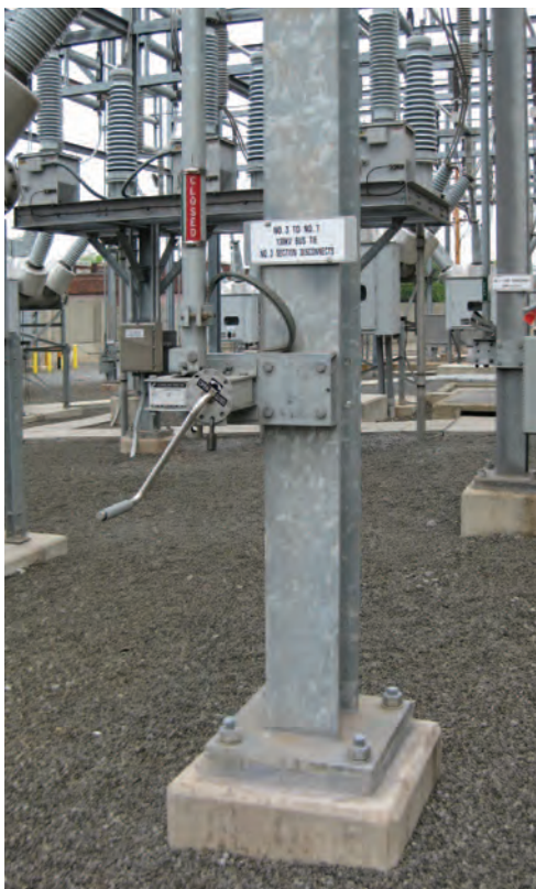
Geared handcrank operator with unbreakable, non-cast stops.
