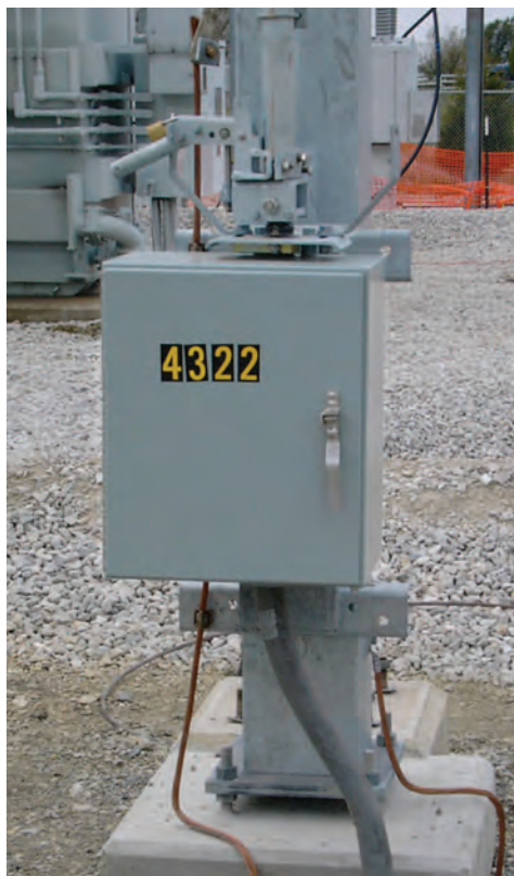
Motor operator type TP-C2 with torque relief decoupler (shown uncoupled).
