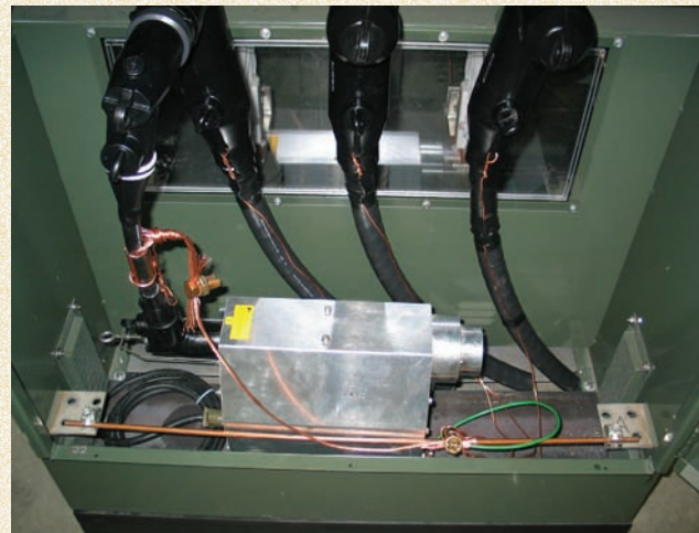
Charging transformer installed in a padmount switch.
