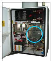
BT-D motor operator with RTU 2000
