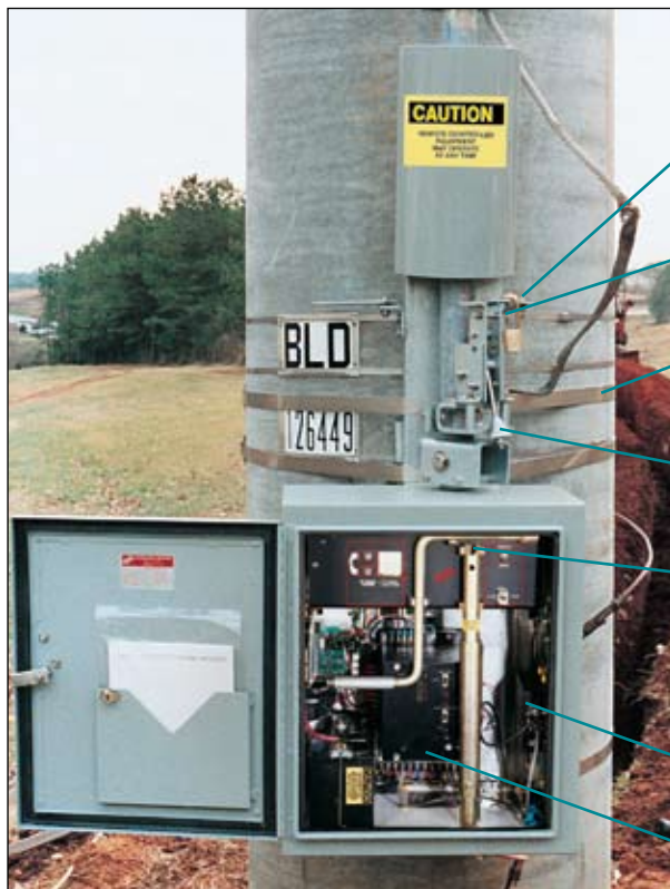
BT-T operating a 115kV SEECO switch.
