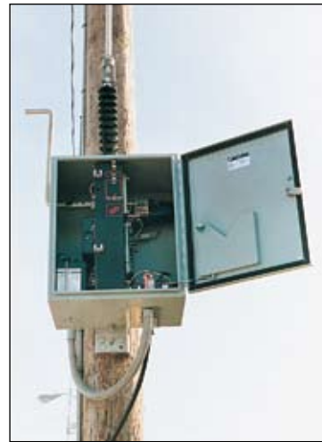
Type BR shows with manual handle in place. Unit is mounted 10 feet above ground.
