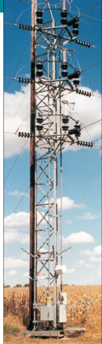
BT-TF motor operator operating a Turner switch.
