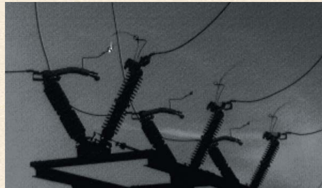
The Polywhip™ interrupter shown on a 138 kV CB-AV switch.
