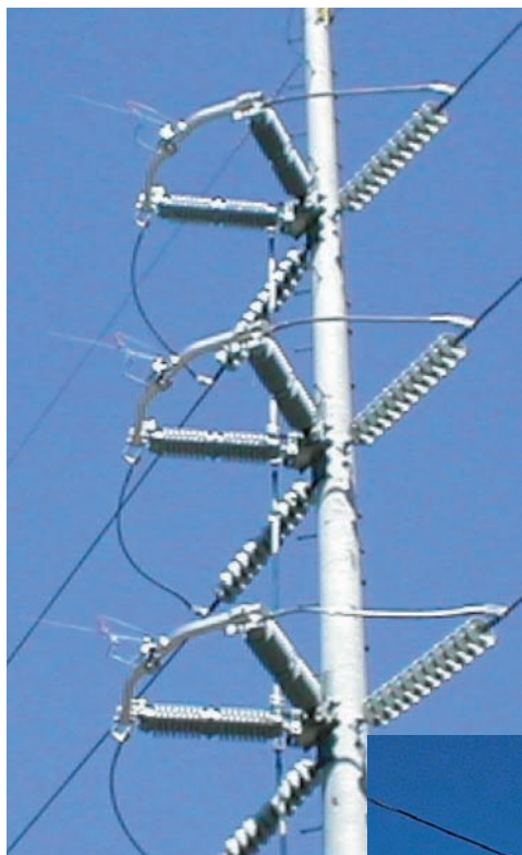
0 ms. Whip contacts are just beginning to separate. A slight spark can be seen.
