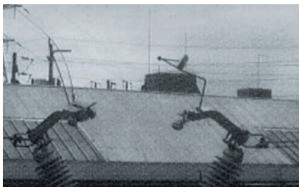
48 ms. The whip has fully opened without re-strike.
